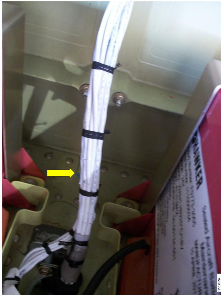
Wire Harness P/N 39-108843 Typical Damage Figure 1
